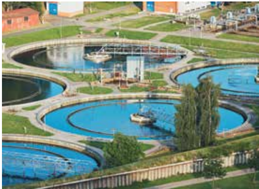
Waste Water Treatment
