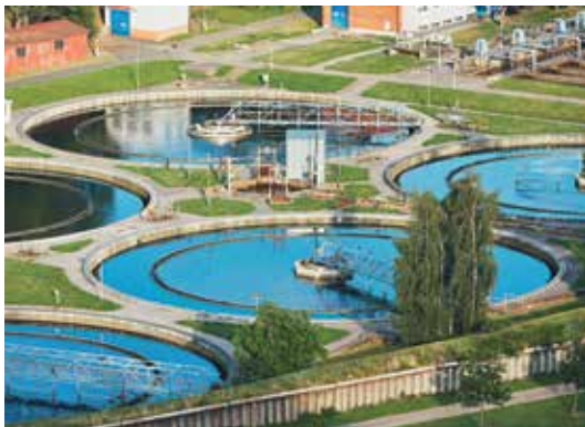
Waste Water Treatment
